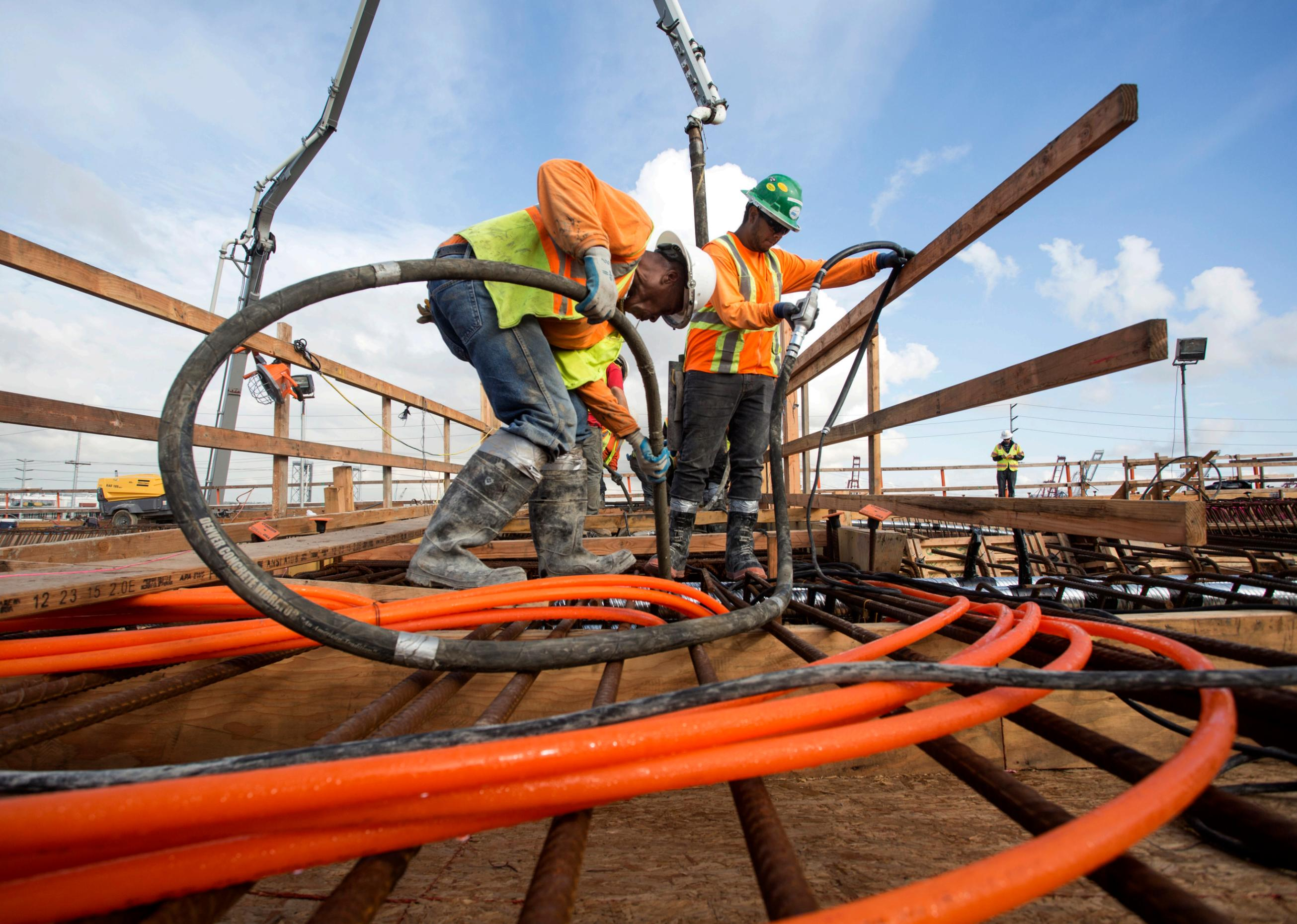
*During a concrete pour of a bridge segment, workers help to complete a clean pour by vibrating the newly placed concrete.*
