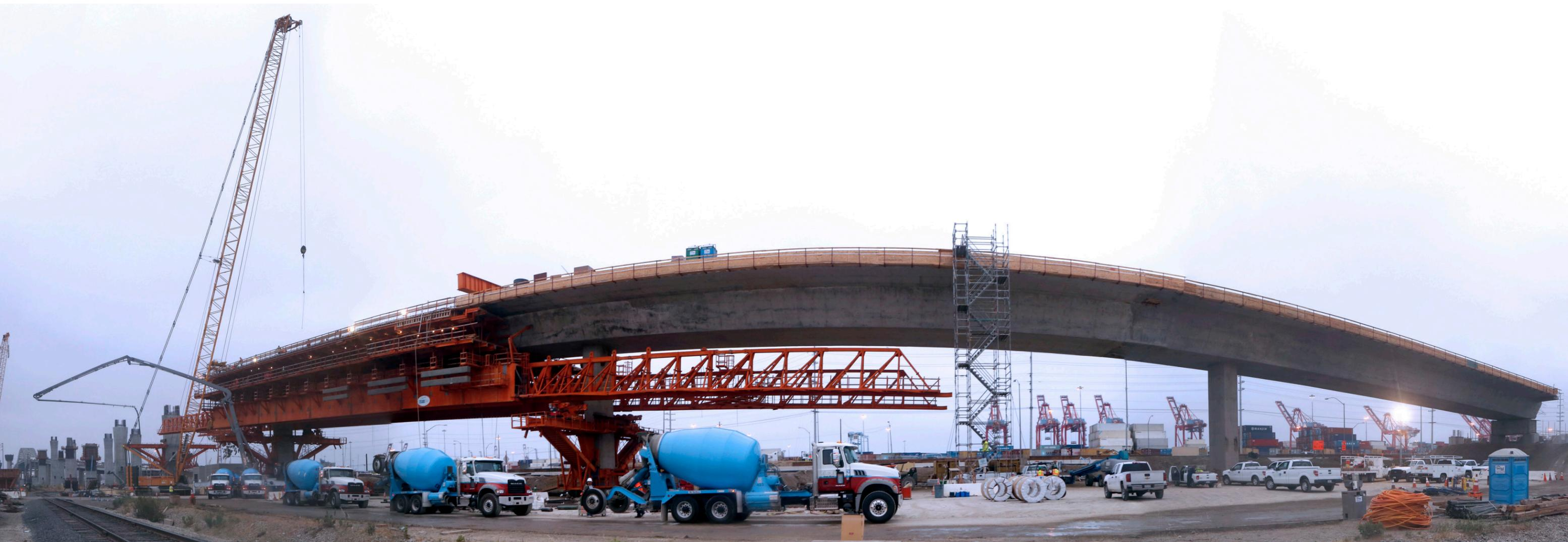
*The orange structure is one of two “Mobile Scaffolding Systems” at the Gerald Desmond Bridge Replacement Project. It is used by bridge builders to provide a form for concrete pours. It helps to save time and material, compared to traditional formwork.*
