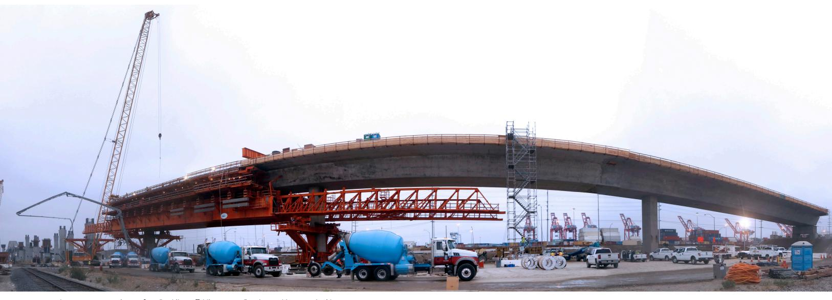
The orange structure is one of two "Mobile Scaffolding Systems" at the Gerald Desmond Bridge Replacement Project. It is used by bridge builders to provide a form for concrete pours. It helps to save time and material, compared to traditional formwork.
