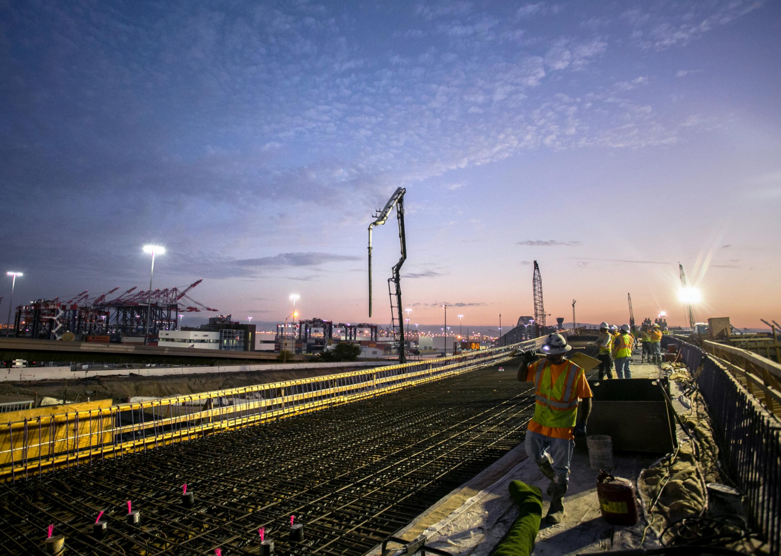
Workers prepare to pour concrete for a new segment of bridge.
