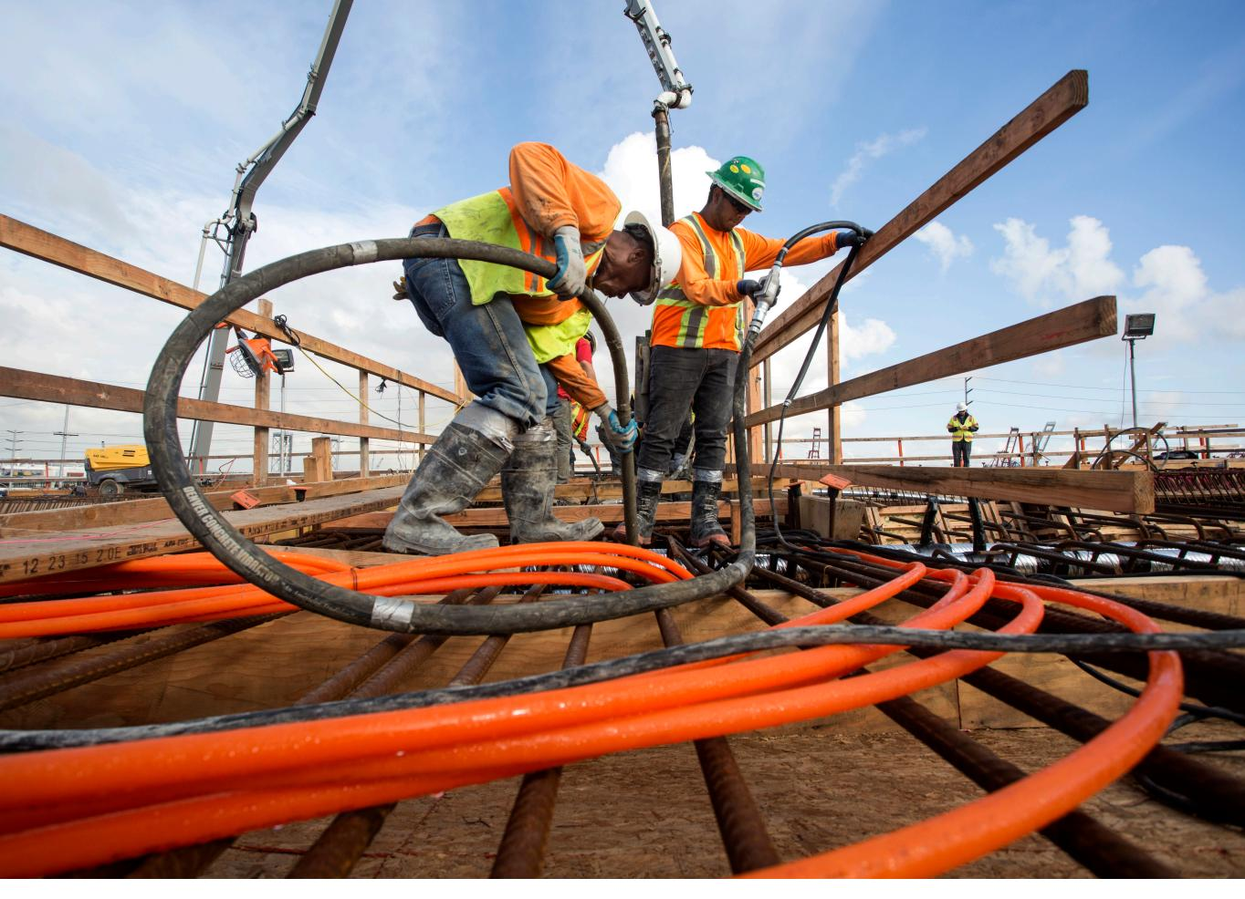
During a concrete pour of a bridge segment, workers help to complete a clean pour by vibrating the newly placed concrete.
